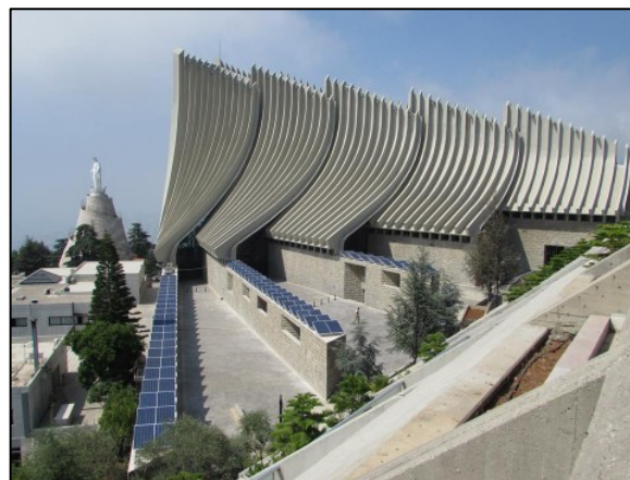
Solar panels on the roof of the famous Maronite Christian church in Harissa, Lebanon. Image: Indevco News Network
